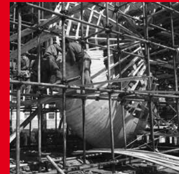
1969 Thin Shell Rib, Monument to Concrete and Steel after completion and during construction in 'Master Builders' Courtyard'
